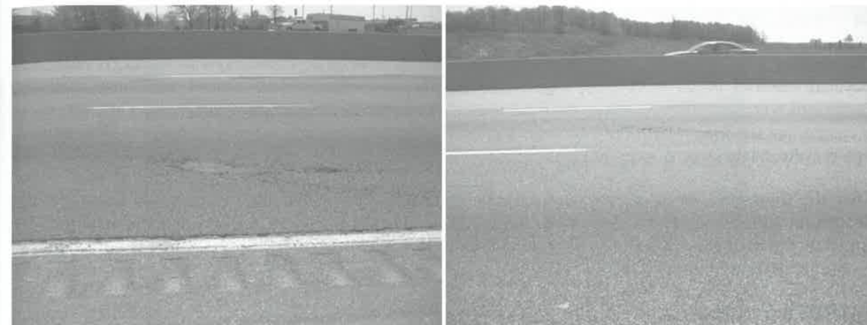
Figure 3. Condition of New DFC Section in 2007 after Eight Years in Service
